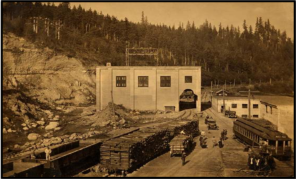
View of the Bull Run Powerhouse, which was completed in 1912.
